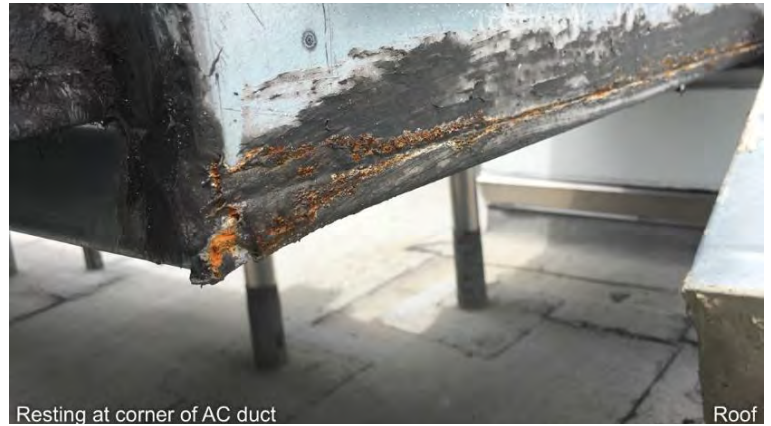
Resting at corner of AC duct Figure 30
